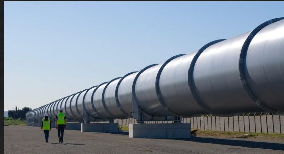
Full-scale Test Track
